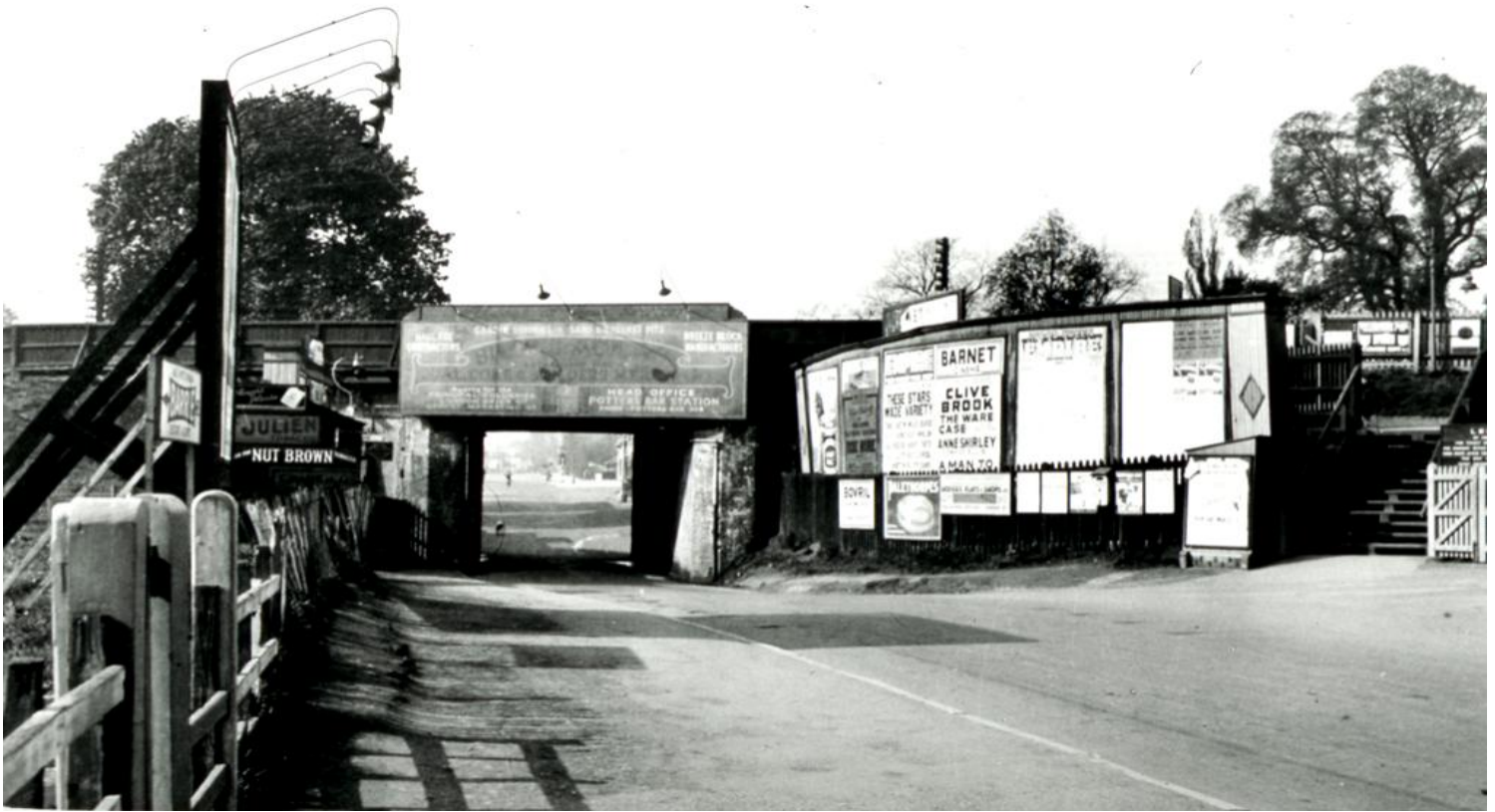
The first Rail Bridge in Darkes Lane Station on Right c1930s, image from the Museum's collection.
